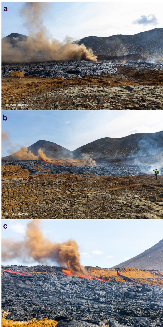
Fig. 11 Lava overtopping of the East Dam on May 22 (courtesy of Elvar Þór Ólafsson). Soil dust plume rose from under the main lava flow over the dam. (a) Seen from the upstream and west of the dam. Heaps HA and HB have been fully overtopped. Only the westernmost end of heap HC is still visible. (b) The overtopping seen from the downstream. (c) Closer view from the downstream of one of the main lava streams at that time and the thick soil dust plume
